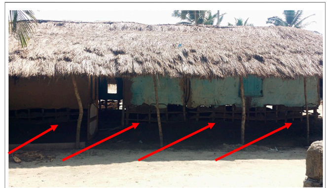
FIGURE 3 | A house in Woarabeba destroyed by the recent flooding even in November 2019 (Arrows pointing to base of the building damaged by flood waters).
